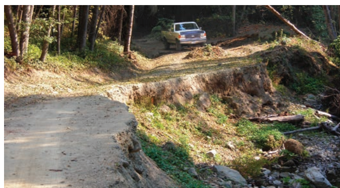
Unpaved roads, especially those adjacent to streams, such as here in the Trinity watershed, often fail after major rain and flood events, adding to erosion and sediment delivery.
